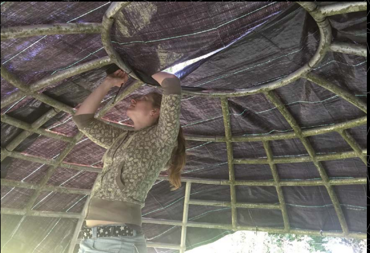
6 Scenographer Katerina Malikova during the building process of the installation space (©2016 Falk Hübner)
